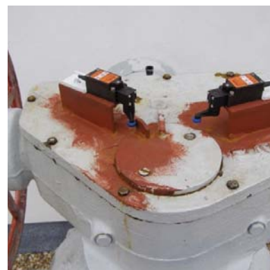
Figure 7. Appli- cation example – valve position monitoring
