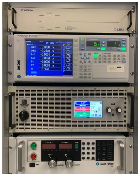
FIGURE 19: EQUIPMENT USED FOR OPERATIONAL TESTING
